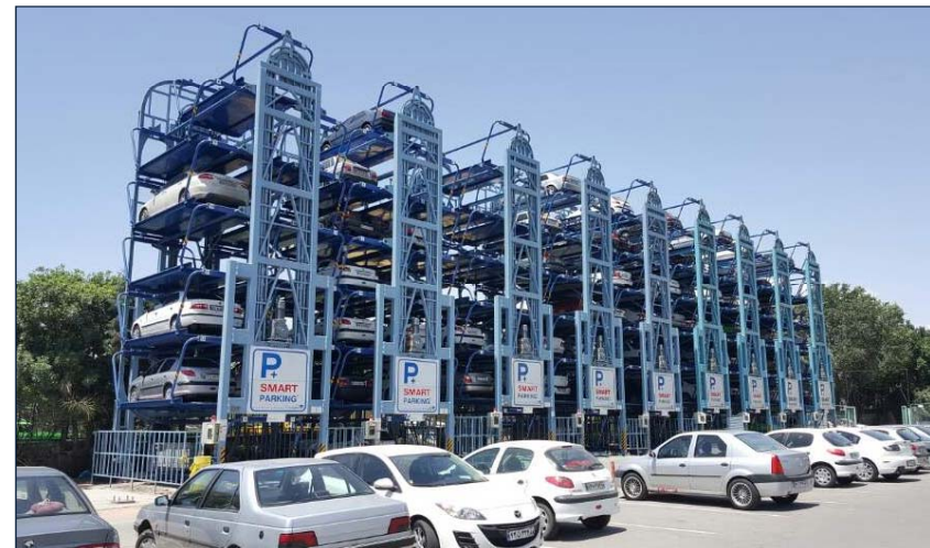
108 car parking lots by 9 units of SM12L, District 15, Tehran
