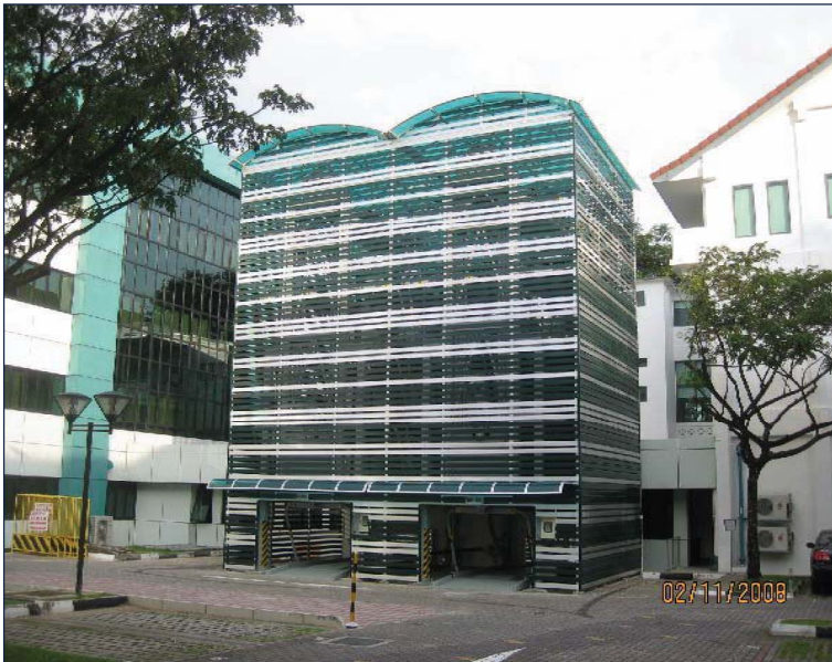
20 car parking lots by 2 units of SM10L, SNEC (Singapore National Hospital), Singapore
